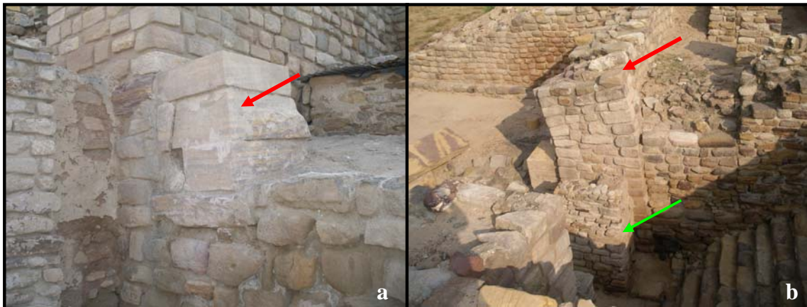
Figure 6. (a) Clockwise rotation of a pillar due to an earthquake 1500 years back at Dholavira Pillar was cracked also, (b) Tilting of walls of Citadel at Dholavira due to earthquake (red arrow) Walls constructed by younger civilization (green arrow)
