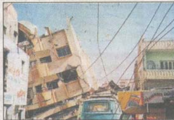
Buildings damaged in 2001 earthquake in Bhuj fort area (file pic)
