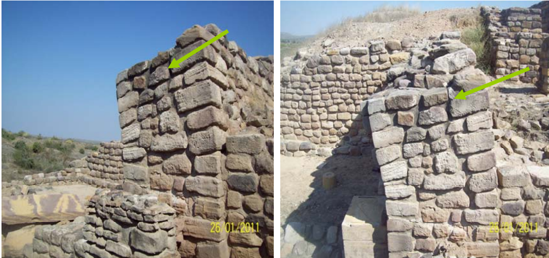
Figure 5: Signature of past earthquake is visible in the form of tilting and rotation of pillars in the North gate of citadel.
